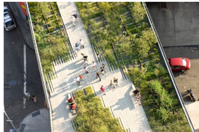
Aerial view High Line
